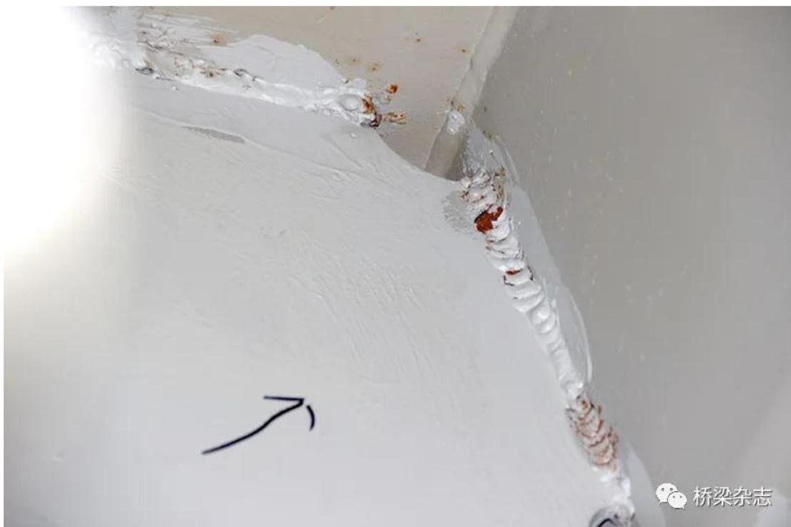
纵隔板与横隔板相交处焊缝开裂锈蚀
